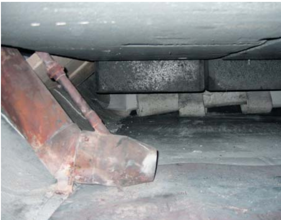
Burner location during baking Fig. 4
